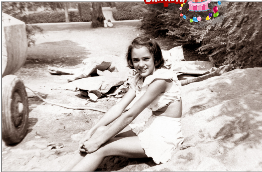
Joan on the pile of sand by the cement mixer in 1949. Her dad was busy plastering the house and rooms in the fall of 1949.
