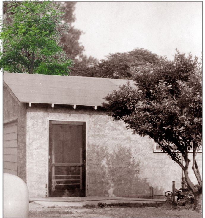
The garage house the Marshes moved into on August 24, 1947. This photo shows the screen door that was added September 13. The exterior had just the first "scratch coat" of plaster.
