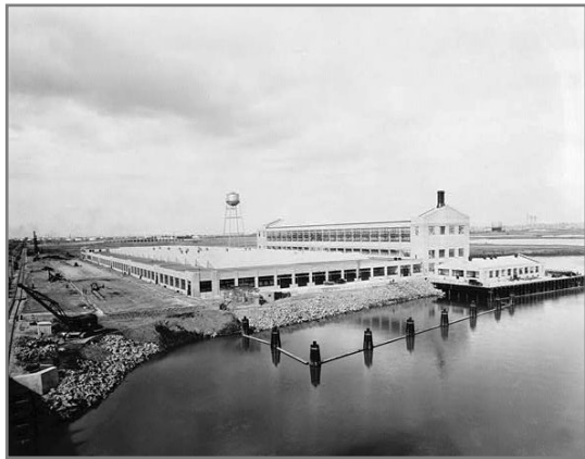
Ford's Long Beach Plant meant a longer drive to work for Lou, so they began looking for a new home to rent.
